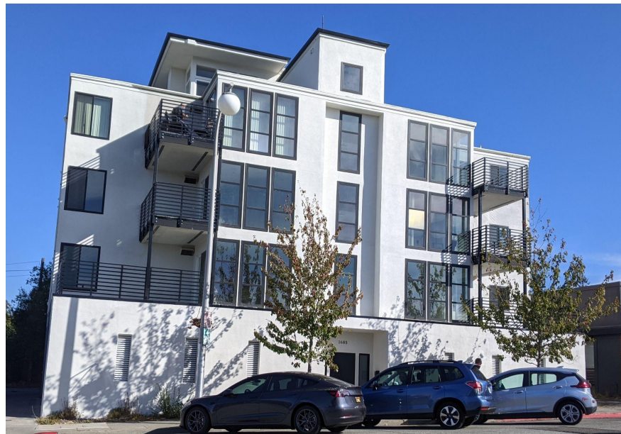
Bay Area CLT Rehab Project
