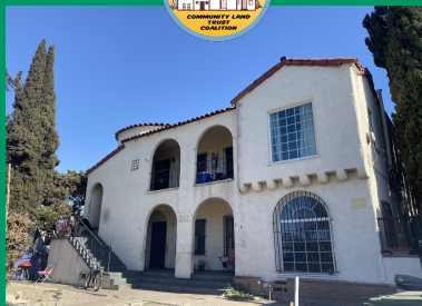
700 Simmons Ave, 11-units, 1930, Unincorporated East LA
